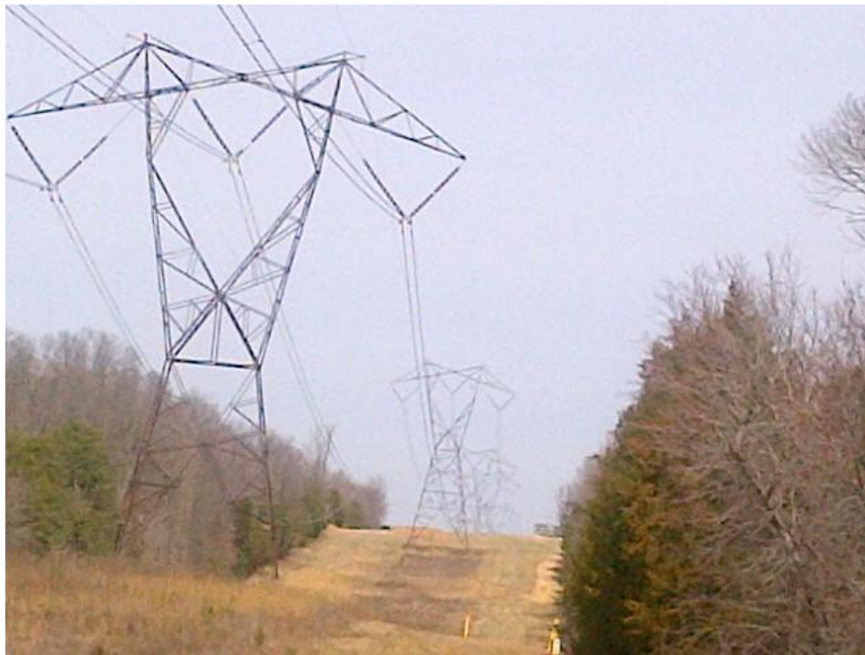
Power Line Structures-South
