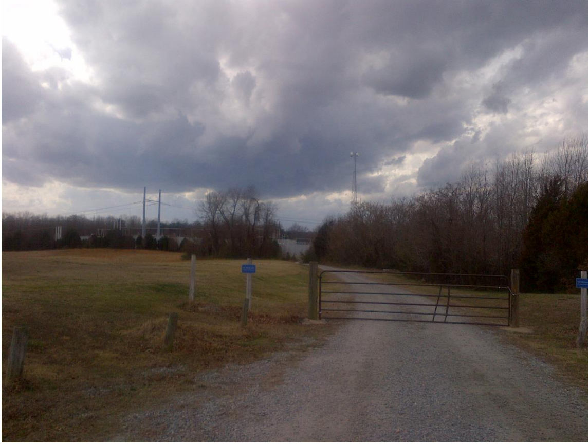
Photo of Sub-station in topographic “Saddle”
