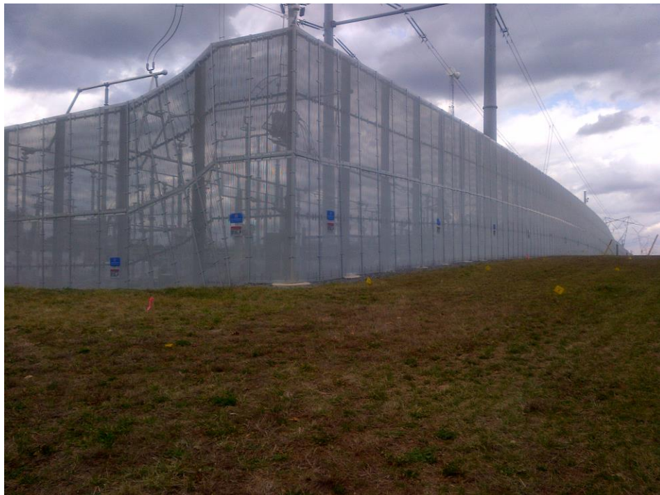
Approximate location of Tower compound
