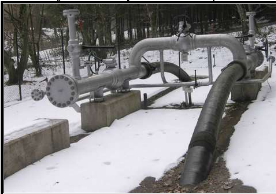
Figure 3: PIG Launcher Site aboveground piping – Please note, proposed fencing will include forest green slats to complete screen the facility.
