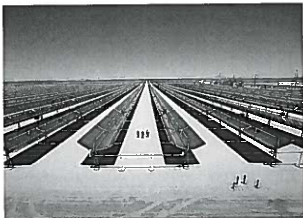
A solar power plant in California's Mojave Desert.
