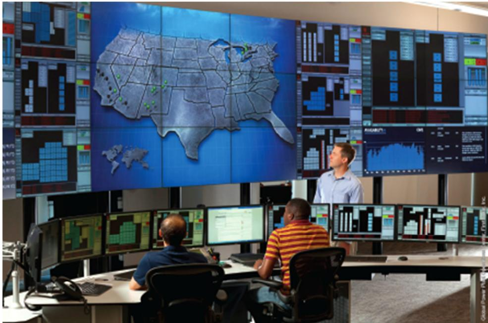
Figure 35: First Solar Operations Center in Tempe, Arizona, from where the company controls over 2,000 MWp of solar power plants operating in the USA [67].
