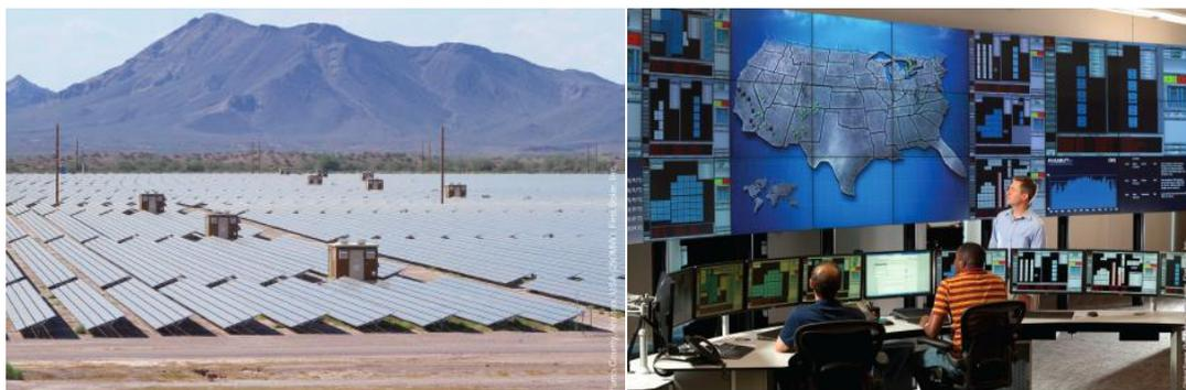
Figure 29 (left): First Solar's Yuma County-Arizona, 290 MWp CdTe PV power plant with grid-friendly plant control and (right) Operations Center in Tempe, Arizona, controlling over 2,000 MWp of solar power plants operating in the USA<sup>69</sup>.
