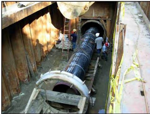
Figure 21: Installation of underground utilities.
