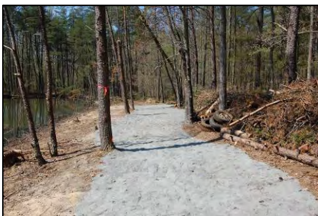
Figure 20: Trailway Construction. Following way marking and clearing, lying down of the trail surface example at the Salamander Loop demonstration trail by the Spotsylvania Greenways Initiative (SGI). In this example stone dust has been used.
